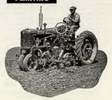
This planter, forward-mounted on a Farmall C tractor, is easily raised by Tauch-Cantrol. Planting depth may be similarly controlled.
